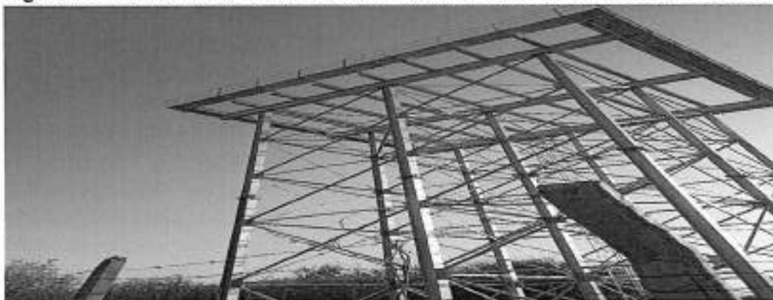
Figure 4: The 15 Meter Tower Where a 300m 3 Steel Tank Was to be Placed
