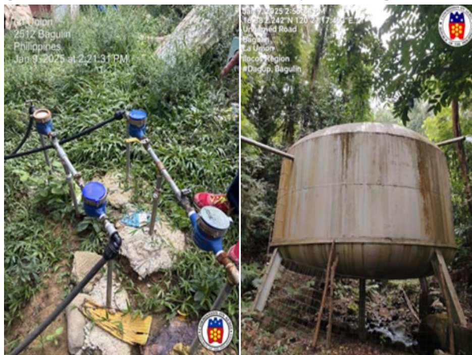
Figure 5: Constructed SALINTUBIG Water System in Bagulin, La Union
